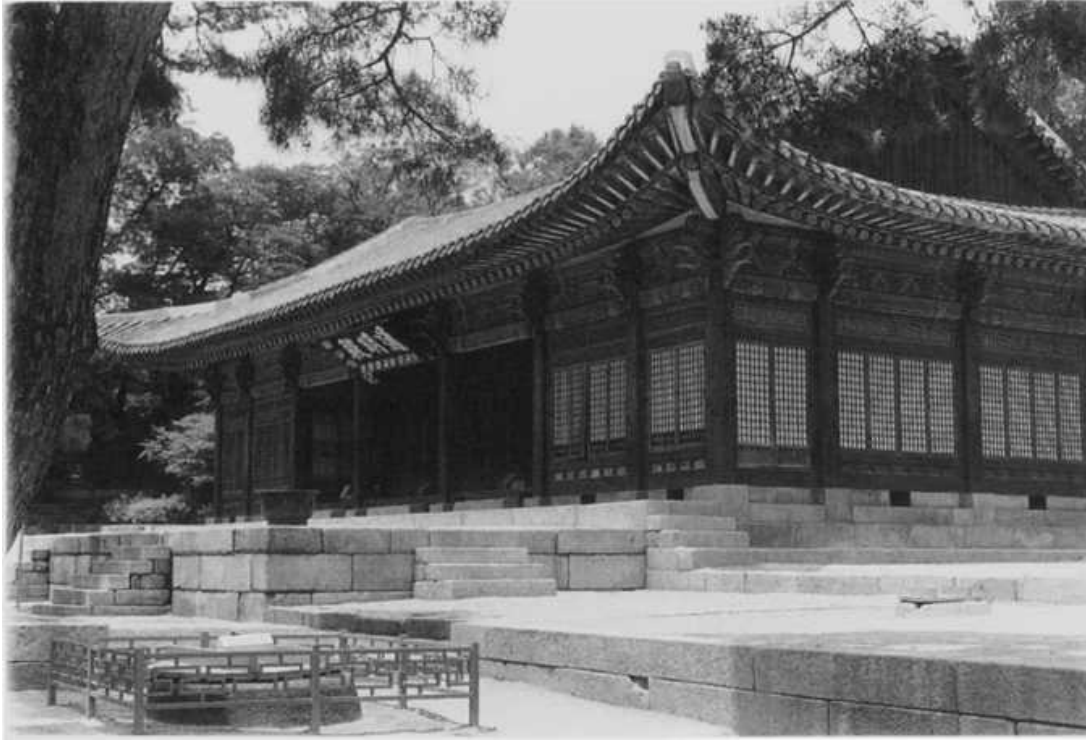
Figure 3. T'ongmyŏng Pavilion in Ch'anggyŏng Palace. It was used for gatherings of either an official or a social nature. It is approximately 40 feet deep by 80 feet wide. The interior consists of one large room.
