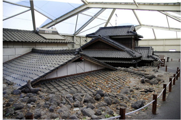
FIGURE 75.18 A number of houses were buried by lahars from Unzen volcano, Japan, and have been covered to protect them from erosion and to make them available to visitors all year round. Photo: P. Erfurt-Cooper.
